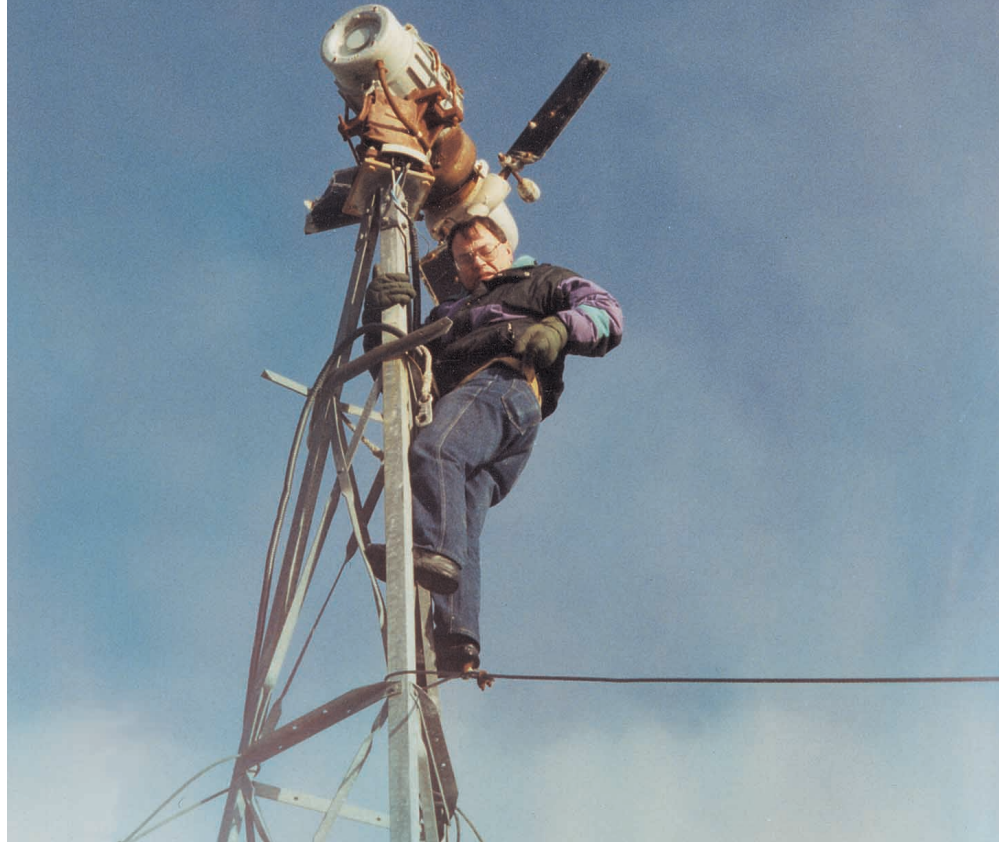
The author prepares to repair a Dunlite BL, 2 KW wind generator that uses a brushless, 3-phase alternator.
